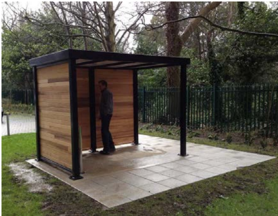
Fully enclosed walls on two sides.
