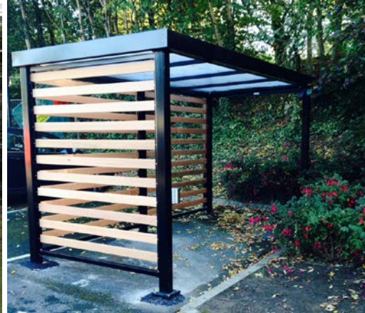
Spacing between boards on two sides.
